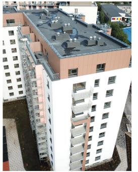
PRO DEV provided several works in Teika, Ropažu Street 14, which included both the interior decoration of the apartment house and the facade work. We installed partitions and plastered walls with plasterboard and painted and also we made tiling works in the bathrooms. In the facade - we made sandwich panels and insulated facade of the building.
